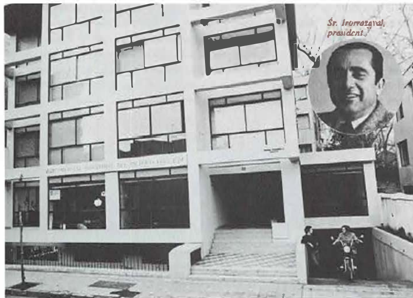
Front view of main office building.
