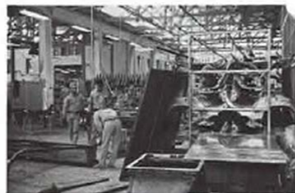
3. Assembled frames are orderly placed on the rack.
