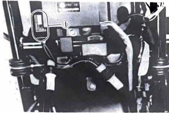
1. CATALYZER control unit
