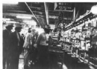
Every work process is smoothly going on
