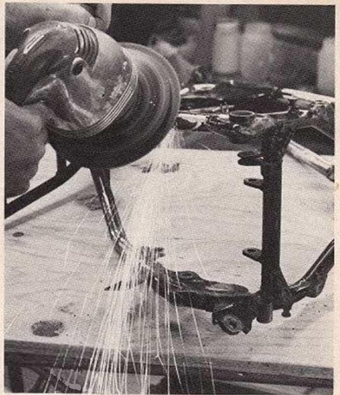
2 By grinding off the old weld, a larger and better welding surface will become available. It will also make for a better looking job.
