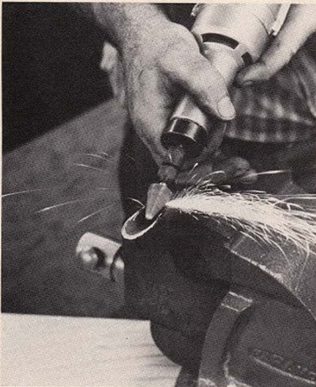
23 The bottom of the new bracing tube should ideally be ground to conform to the bend of the frame member. Protect your eyes from the sparks.
