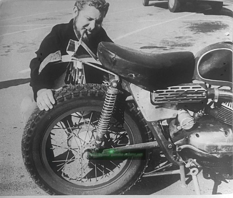
Wiggle rear wheel back and forth to check for swing-arm-bushing wear.
