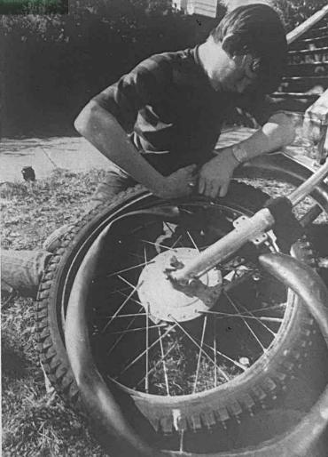
If there is no water handy inflate the tube and 'feel' for the leak with the cheek. If the leak can't be located, blow the tube up some more, about twice natural size.
