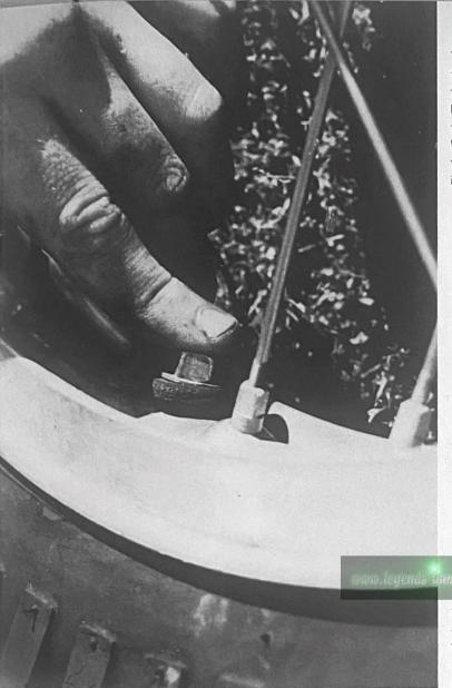
The trick in installing security bolts is to tuck them haphazardly under the bead and then push them up into the tire to the full length of their bolts. Put a little air in the tube and the bolt will settle into position. Wiggle it a bit to make sure and then inflate the tube. Tighten the nut after the tire is inflated.
