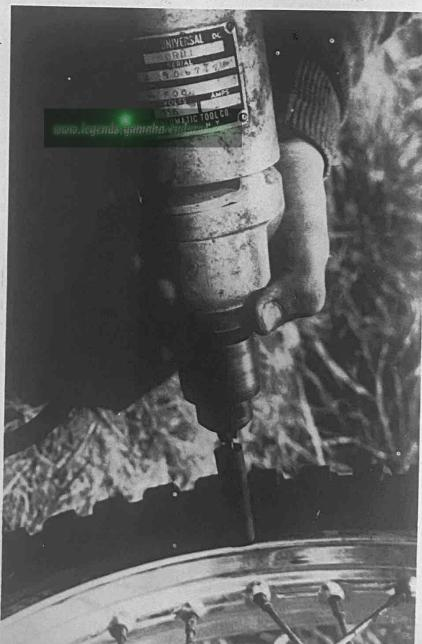
The drill stop in use — without some means of stopping the drill it will probably go clear through the casing into the tube when the bit 'breaks through' the rim!
