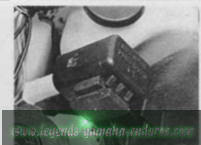
11.1a The turn signal relay is situated between oil and expansion tanks on TZR model ...
